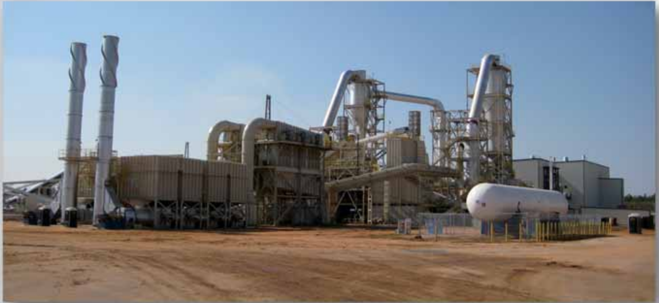
Green Circle Pellet Plant, Florida
